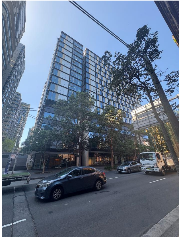
Figure 1: 6 Central Park Avenue, Chippendale, viewed from the west
